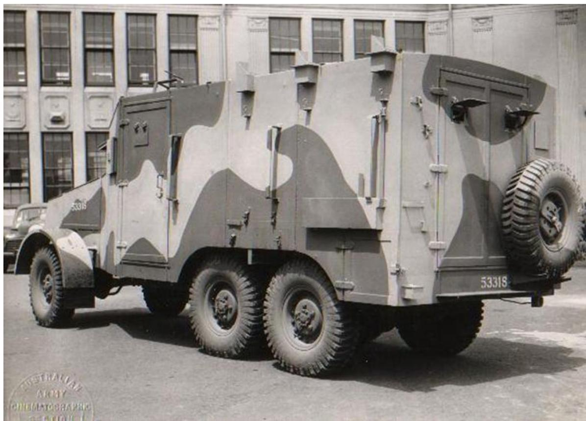
**The ACV showing the rear door, the spare wheel mounting and mounts for the radio aerials**
