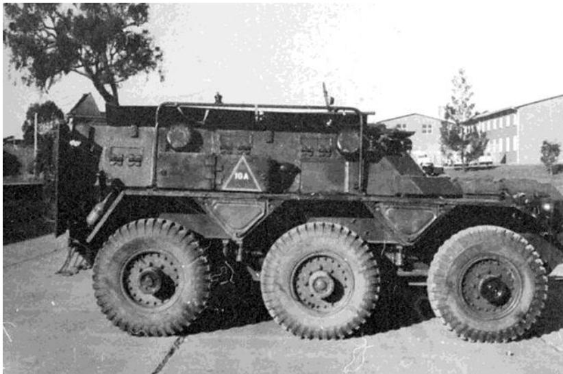
**The Saracen Command Vehicle showing the reduction in height of the vehicle when the turret was removed.**
