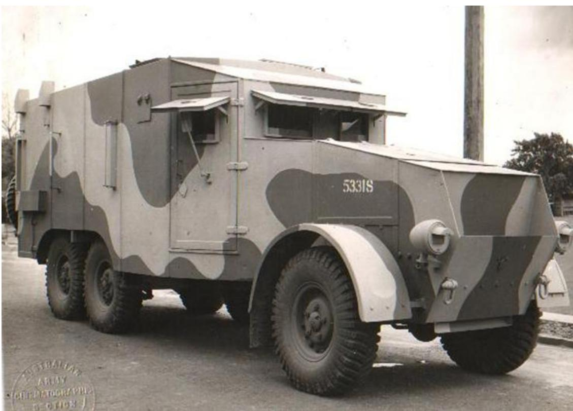
**A view of the ACV showing the radiator scoop and the openings for the driver's compartment.**
